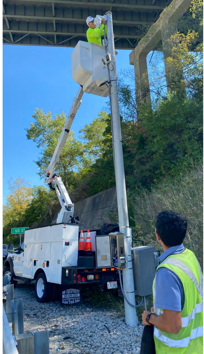
Installation of traffic counter on I-275
