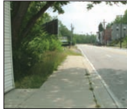
Pedestrians are forced into the roadway when sidewalks end abruptly.
